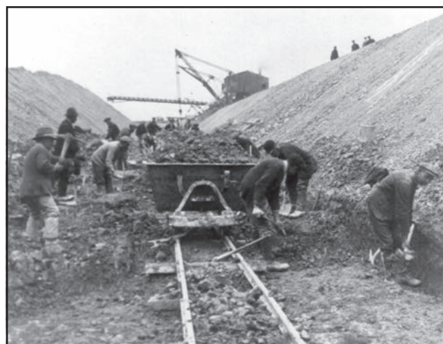
Figure 8. Coprolite diggings at Trumpington, Cambridge, during World War I, with an early dragline in the background (photo: Cambridgeshire Collections).
